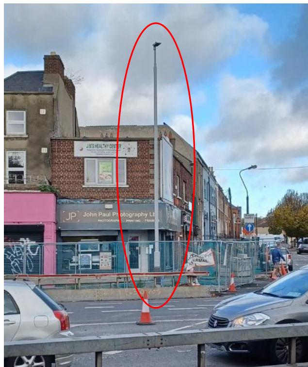
Fig. 3 – Embellishments yet to be installed (bottom of Fairview Avenue Lower)
